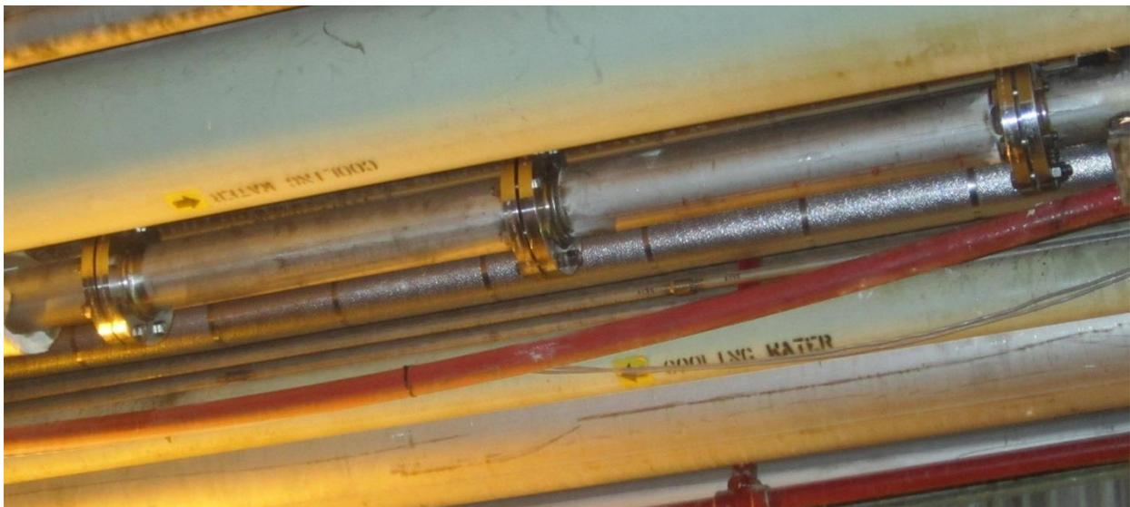
*Contaminated and clean 30" [762mm] pipe spool sections*
