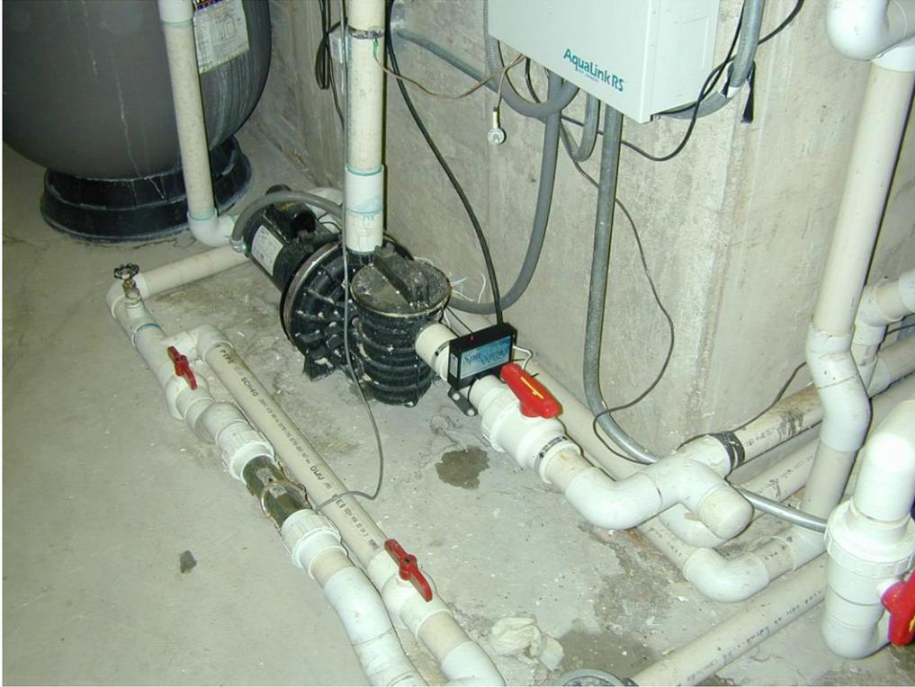
Photograph of installed *HydroFLOW* water conditioner
